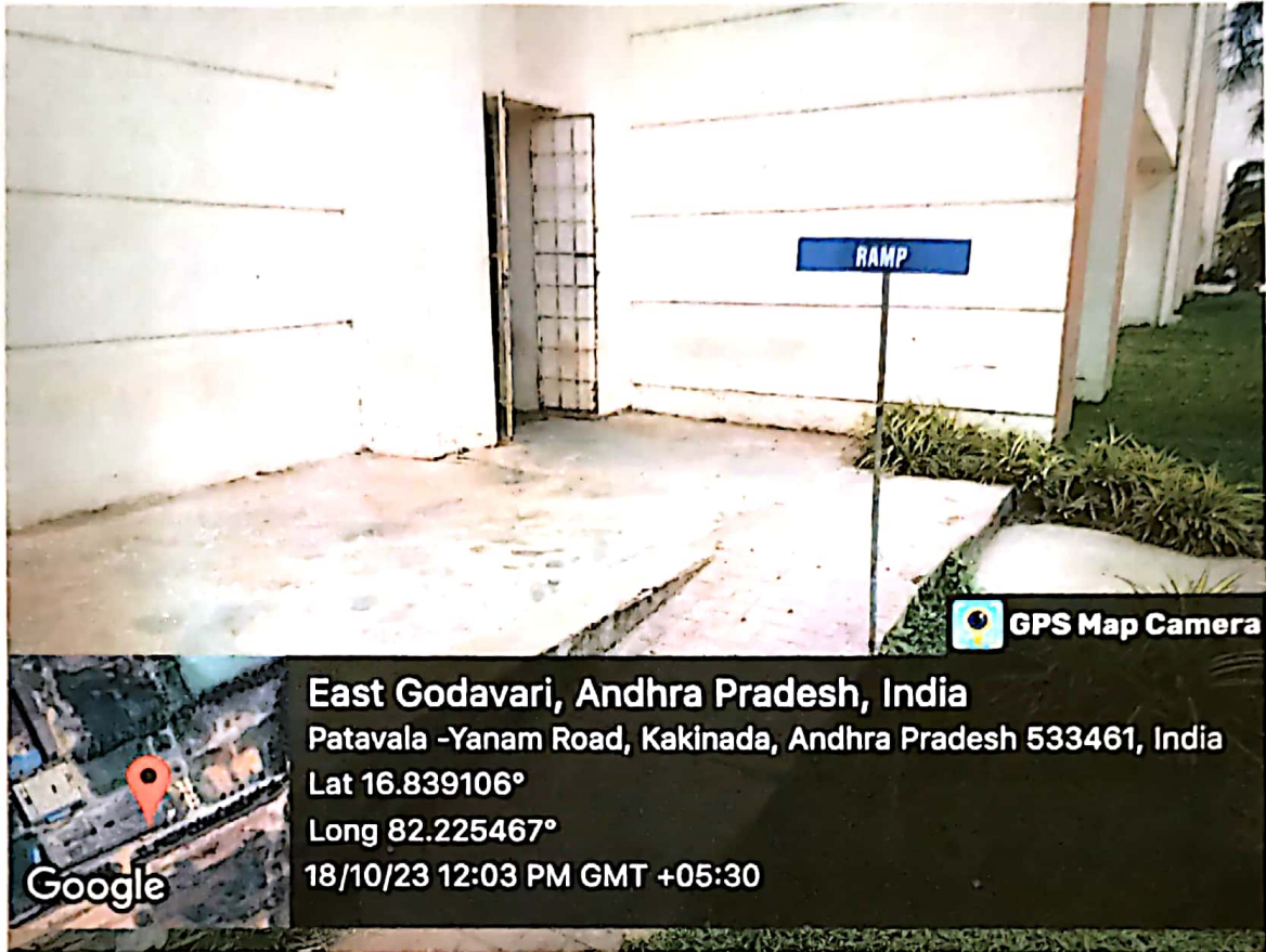
Picture of Ramp
